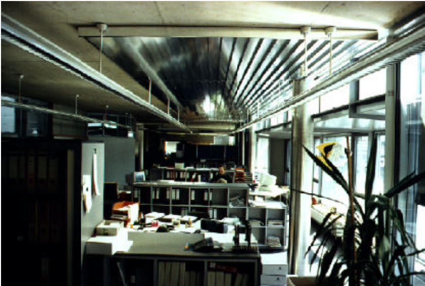
Office in the ground floor, the strip windows under the ceiling contain lightguiding glass to reflect sunlight to the mirrors under the ceiling. This system enhances the daylight penetration on sunny days significantly.
